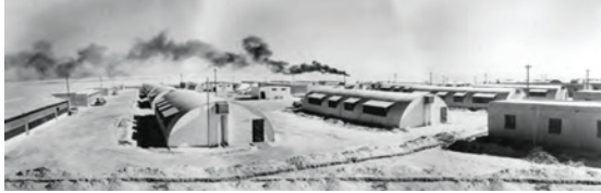
Figure 6: The steel prefabricated Nissen hut structures shipped from Abadan and London. (Source: BP Archive.)
