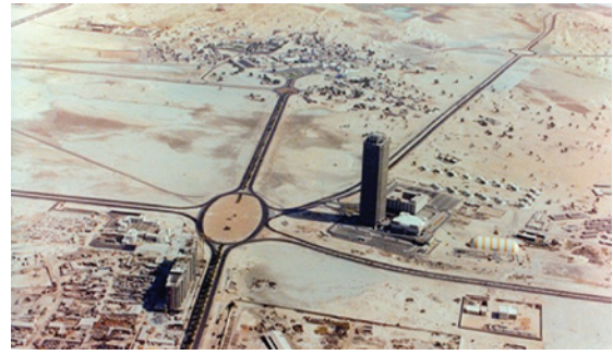
Figure 19: Dubai World Trade Center, Dubai. (Source: Dubai Museum Archive.)
