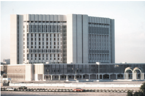
Figure 18: Dubai Hospital, Dubai 1974. (Source: MIT Library.)
