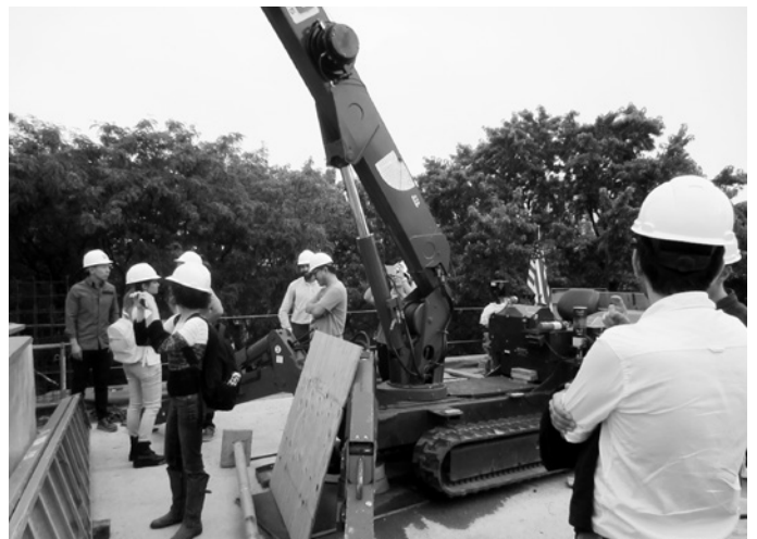
Visit to Tadao Ando- designed Wrightwood 659 under construction, September 23, 2016. (Led by Daniel Whittaker.)
