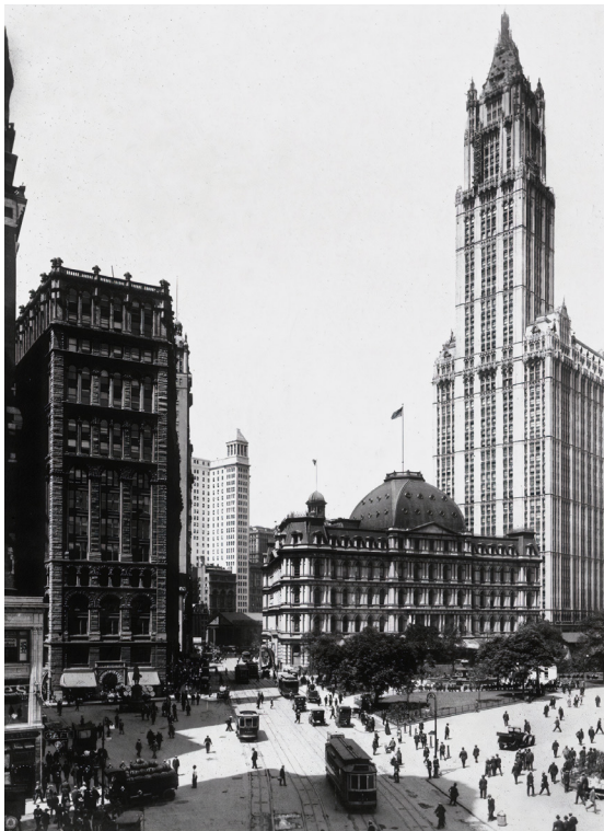
Woolworth Building on City Hall Park at Park Row, New York. Photographer unknown, ca. 1915. Prints & Photographs Division, Library of Congress.
