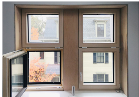
Figure 3: Window configuration. Left bottom window is engaged, with a smart sensor on the window bench.
