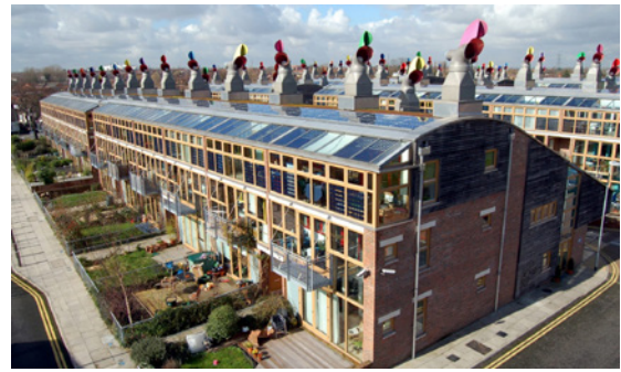
Figure 2: Solar PV on the roof. (Source: BioRegional, 2016.)
