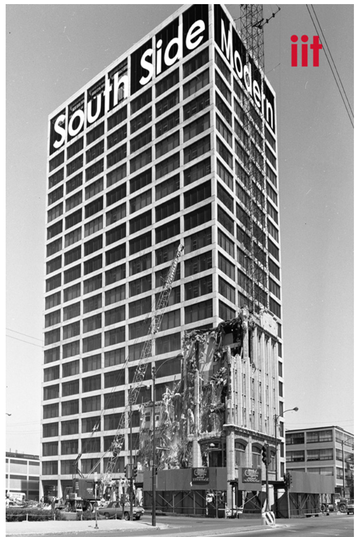
IITRI Tower, Schmidt, Garden & Erickson, circa 1965 + Binga Arcade. Photo courtesy of IIT University Archives and Special Collections.
