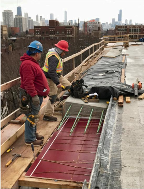
Figure 12: Forming soffit drip edge.
