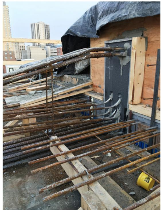
Figure 8: Thermal break at reverse corbel supporting upturned beam.
