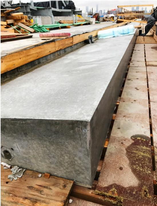
Figure 13: As perfect as possible: Flat fascia and cold joint at cantilever.
