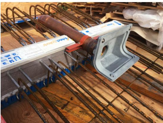
Figure 7: Schöck Isokorb with drain.
